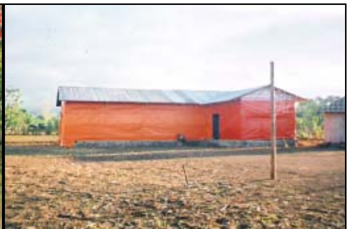
Kam Butter church urgently needs more repairs
